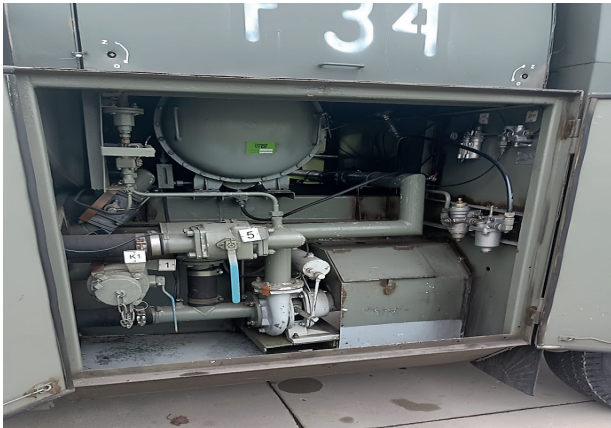
Fig. 6. Fuel installation on the CD-7.5 B tanker-dispenser
